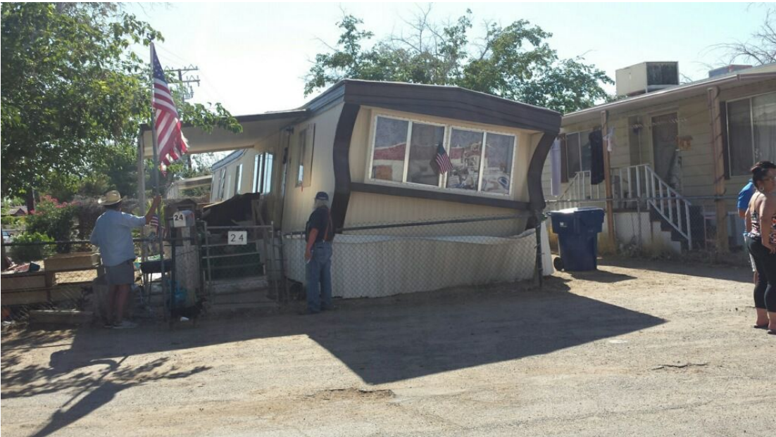
Damage to a mobile home in Ridgecrest, California in Thursday's M=6.4 earthquake. Photo courtesy of bakersfield.com .
