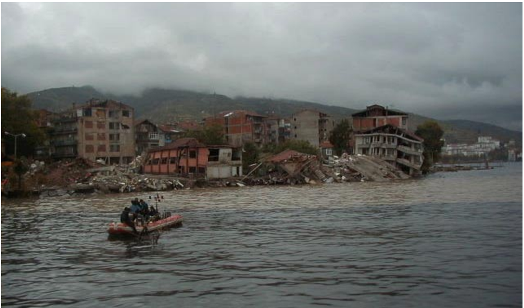
Figure 3.3. At Cinarlik Park near Degirmendere (location 21 in figure 3.2.), a hotel, restaurants, shops, and trees along the shoreline subsided into the sea, at the place where the seawater changes to a lighter color. The divers on the boat were looking for a car dragged into the sea by the wave.
