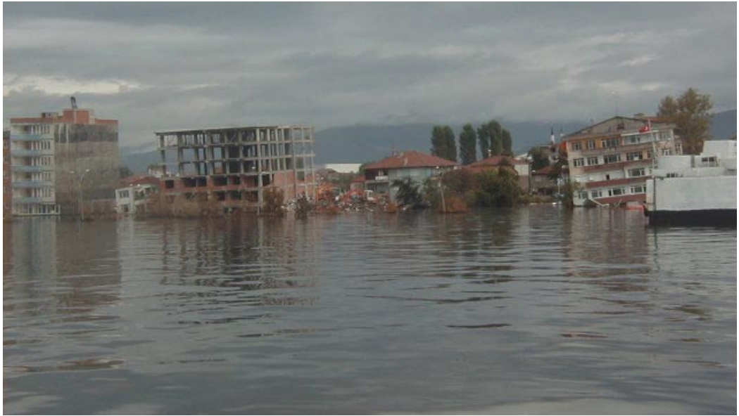
Figure 3.4. A view from the sea of the subsided coastal area at Kavakli, west of Gölçük (location 20 in figure 3.2).
